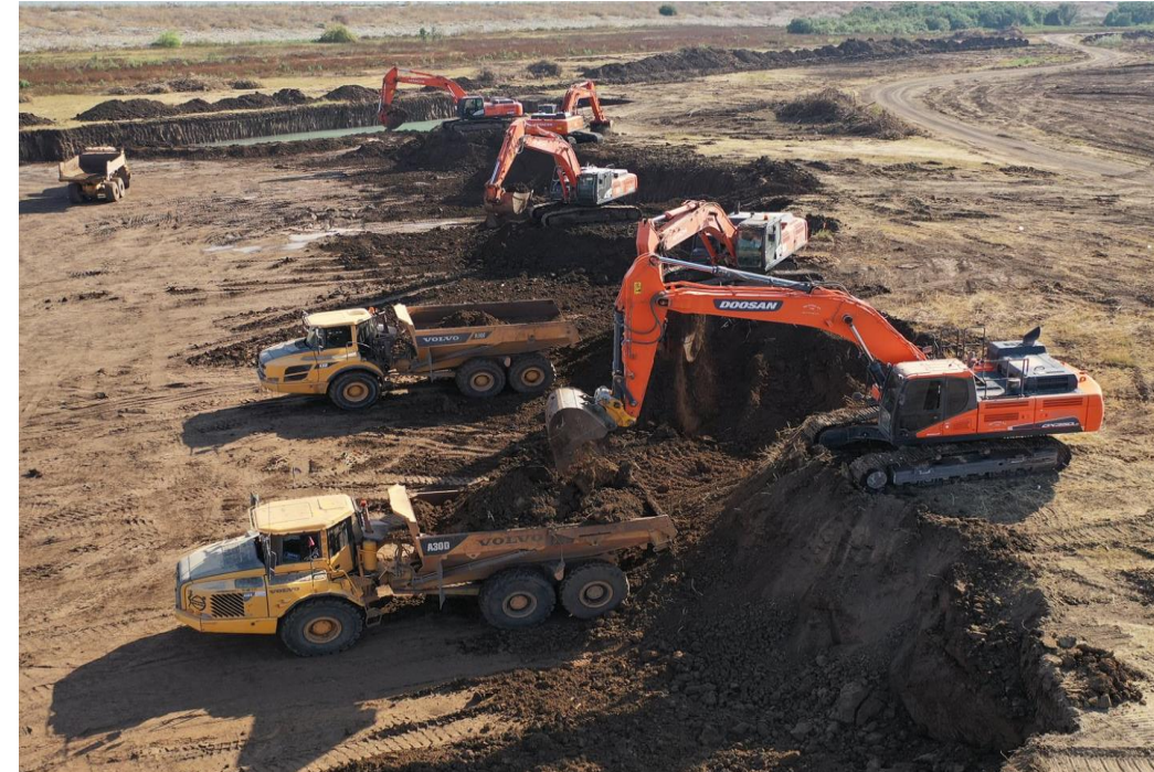
Sediment Removal from Baruch Reservoir 2022
